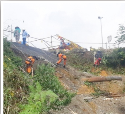
Sod Facing Site Geothermal Drajat II, Garut
