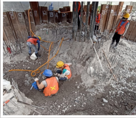
Demolition Pile Cap SCTV Tower, Surabaya
