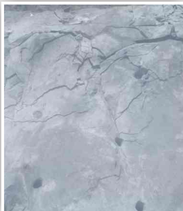
Quarry andesit, Tegal
