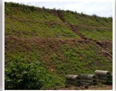
Hydroseeding Kulawi, Palu
