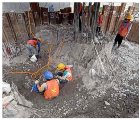
Demolition Pile Cap SCTV Tower, Surabaya
