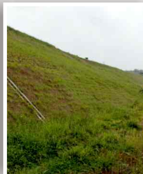
Hydroseeding, Toll Cisumdawu, Jawa Barat
